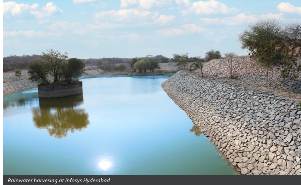
Rainwater harvesting at Infosys Hyderabad
