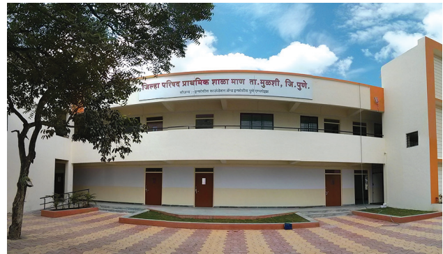
The newly-constructed classrooms under the MySchool program of Pune DC CSR team
