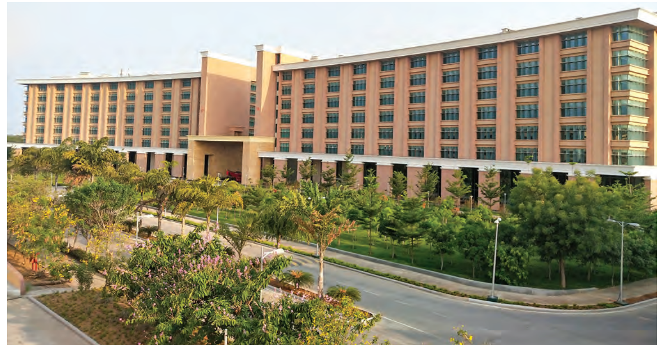
LEED Platinum-rated building in the Infosys Hyderabad SEZ campus
