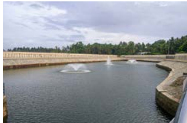
Rainwater harvesting pond in Infosys, Thiruvananthapuram campus
