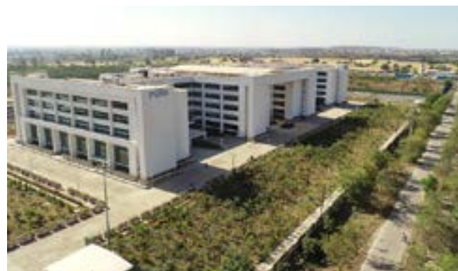
Infosys, Indore SDB – LEED Platinum certified building
