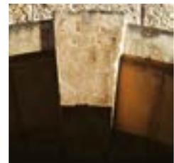
A keystone is the wedge-shaped stone placed in the middle of an arch. The other elements in an arch depend on this architectural foundation as it connects the sides together and distributes the weight down the sides. Without the keystone, the arch would collapse.
