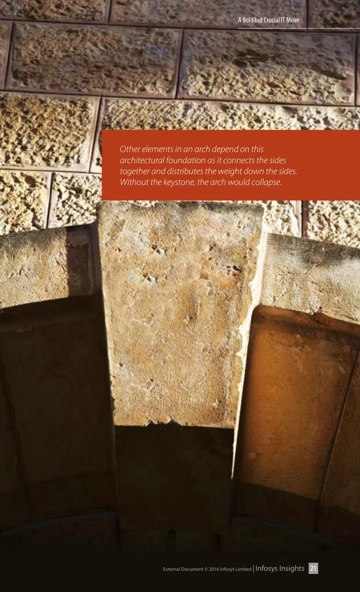
*Other elements in an arch depend on this architectural foundation as it connects the sides together and distributes the weight down the sides. Without the keystone, the arch would collapse.*
