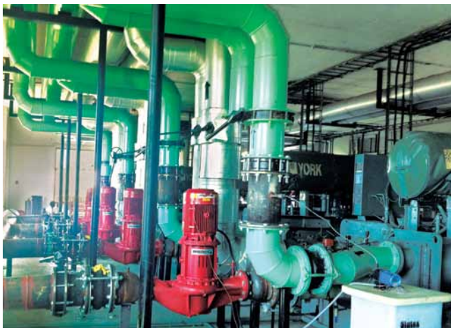
Figure 5: End-suction pumps – before retrofit
