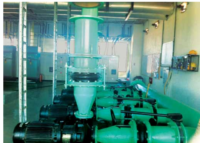
Figure 6: In-line pumps – after retrofit
