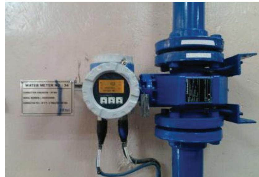
Smart water meter for online monitoring of water consumption
