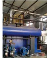
**Hybrid briquette-fired boilers** for steam generation; 90% reduction in refractory, up to 40% reduction in footprint, and fuel flexibility between biomass and fossil fuels
