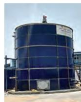
**Waste-to-energy biogas plant with 1-ton capacity**, at full operational capacity, can generate up to 25KW per hour electricity
