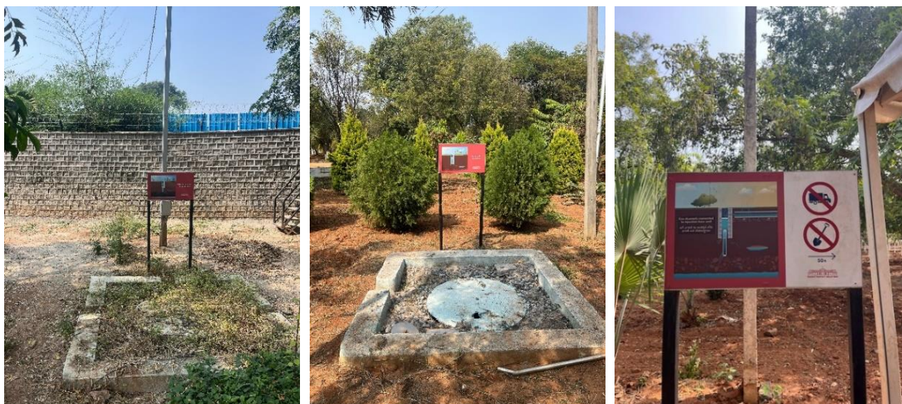
Figure 213: Injection borewell (Left), Recharge pit (Middle) and Board depicting the placement of eco-channel (Right)
