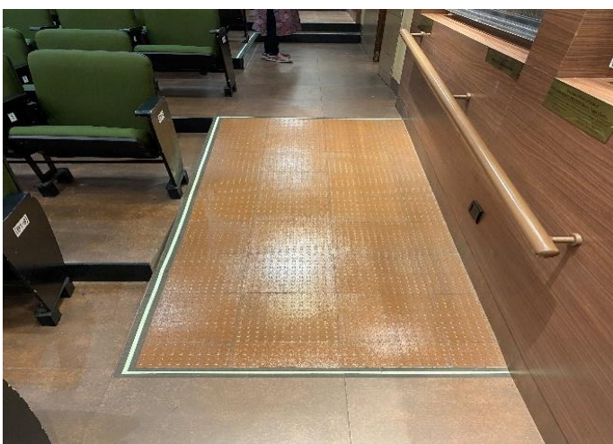
Figure 153: Ramp Constructed to Enhance Accessibility
