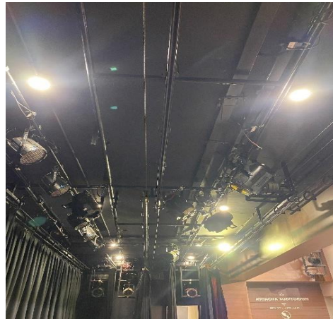
Figure 146: Newly Installed Lights
