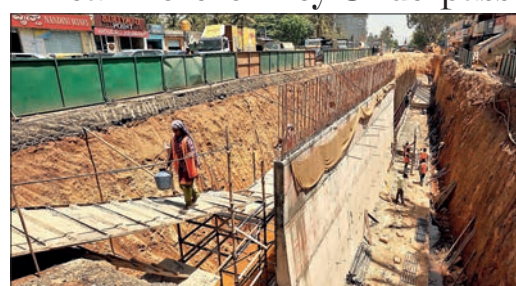
The work on the underpass at Kundalahalli junction, conceived a decade ago as part of a signal-free corridor and expected to reduce traffic congestion towards Hope Farm Junction, has picked up pace. But BBMP officials say the project will take at least a year to complete. — NARASIMHA MURTHY
