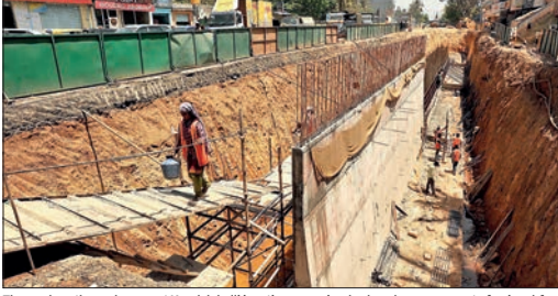
The work on the underpass at Kundalahalli junction, conceived a decade ago as part of a signal-free corridor and expected to reduce traffic congestion towards Hope Farm junction, has picked up pace. But BMRC officials say the project will take at least a year to complete. — NARASIMHA MURTHY
