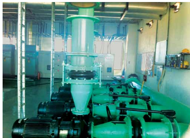
Figure 6: In-line pumps – after retrofit
