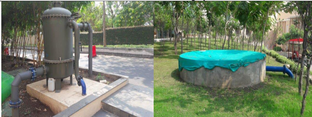
Rain water harvesting system
