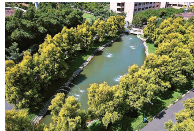
Rainwater harvesting pond in Infosys, Bengaluru campus
