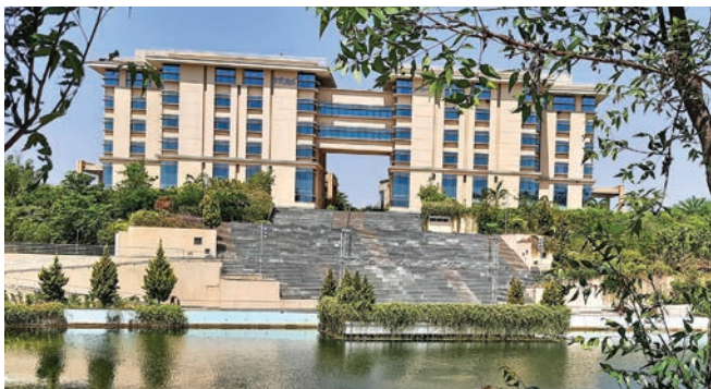
Infosys, Hubballi SDB - LEED Platinum certified building
