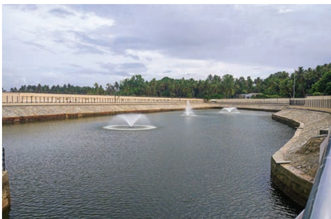
Rainwater harvesting pond in Infosys, Thiruvananthapuram campus
