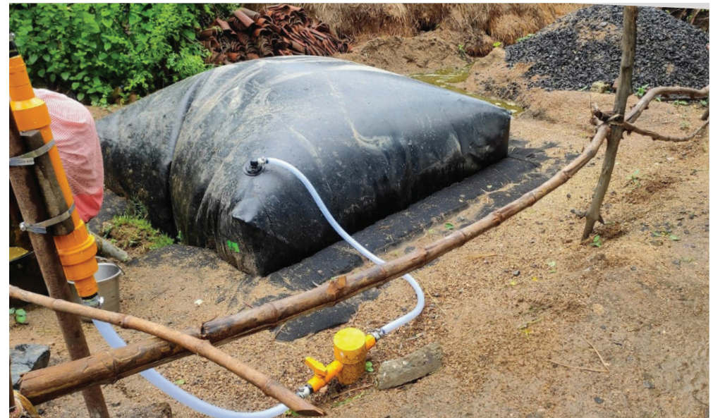
Self sustained Biogas unit
