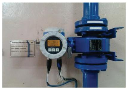
Smart water meter for online monitoring of water consumption
